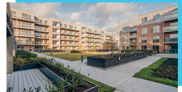
■ Respond Housing at Elanora Court, Longmile Road, Dublin 12
